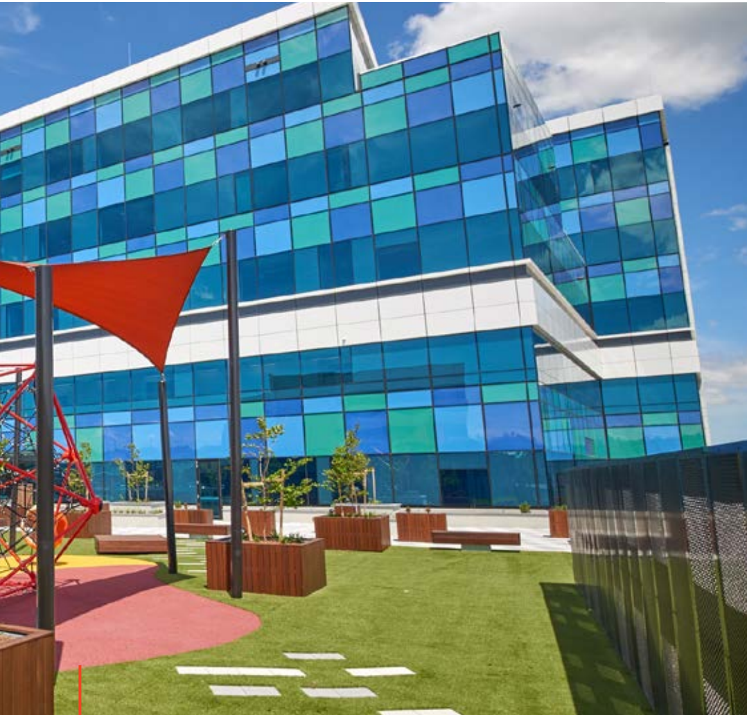
Pictured: The new St John of God Berwick Hospital opened on 18 January 2018..
